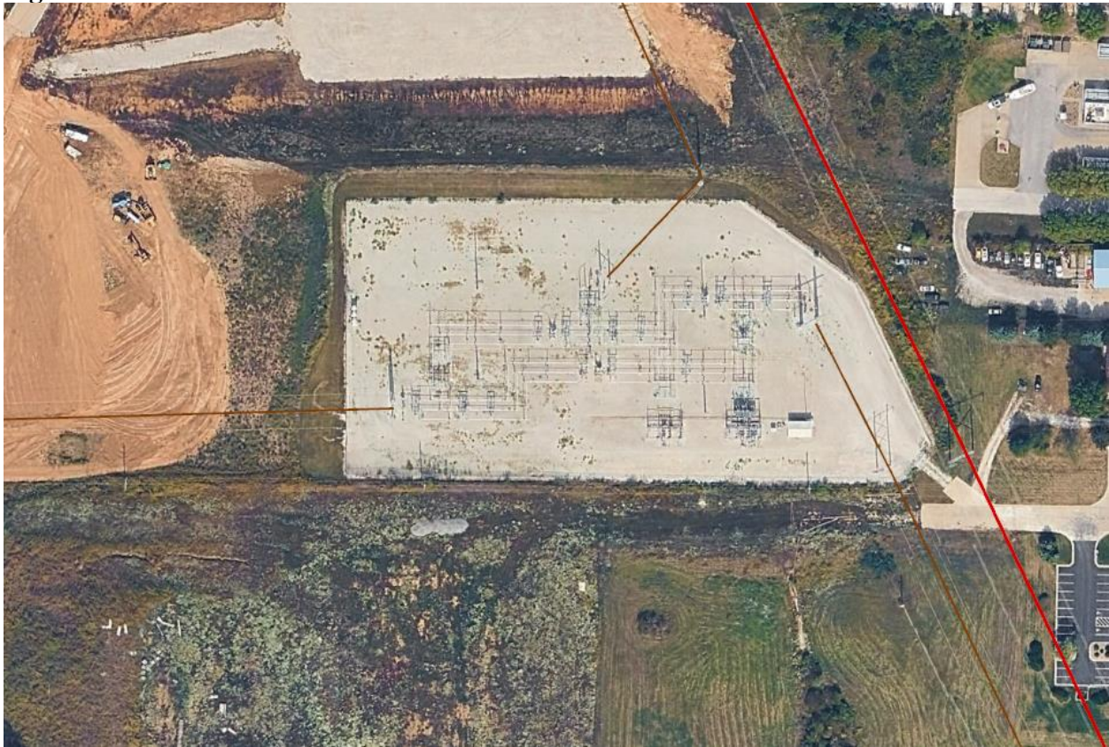
Figure 1 – Smithville 161kV Substation
